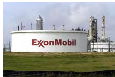
Exxon Mobil Corp. has begun construction on a new production unit at its polyethylene plant in Beaumont, about 80 miles east of downtown Houston.
